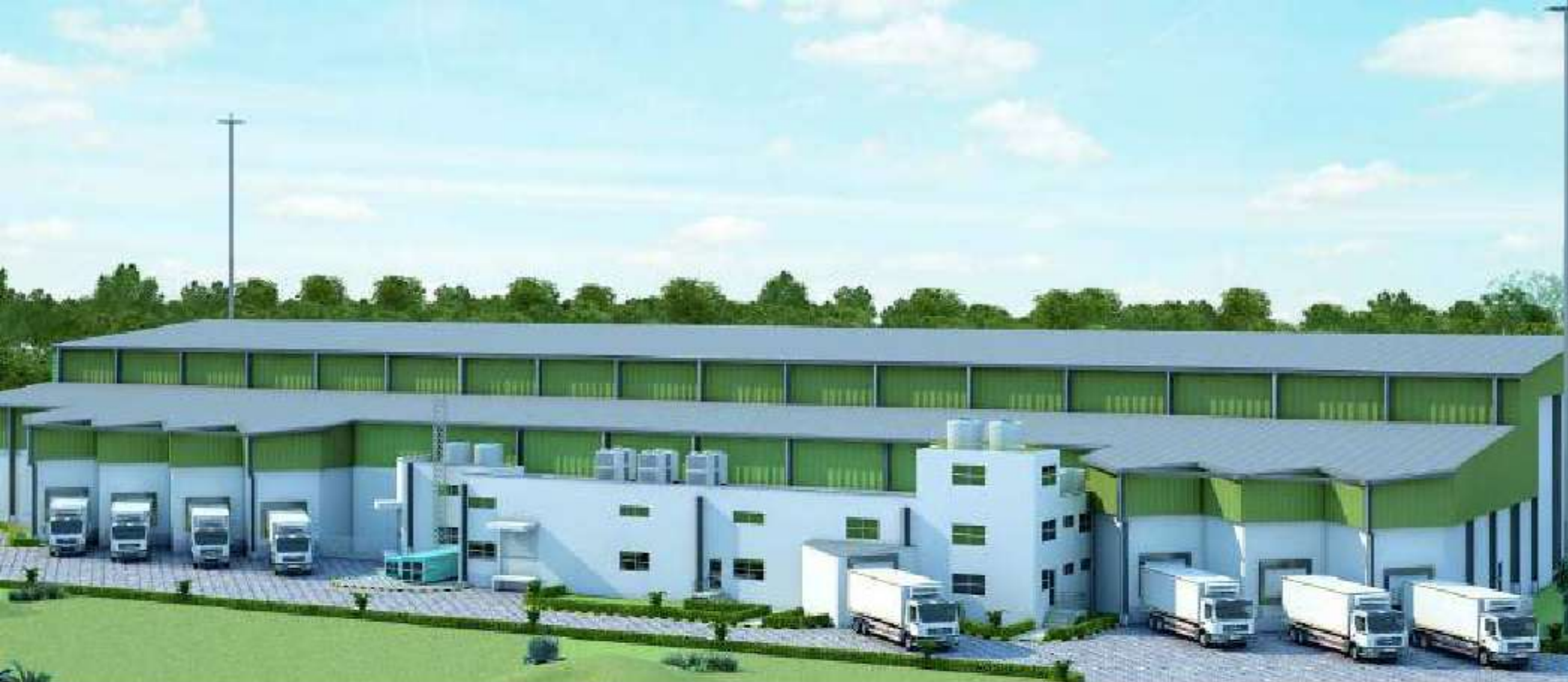
HIND Terminals, Cold Warehouse, Prithla, Haryana
